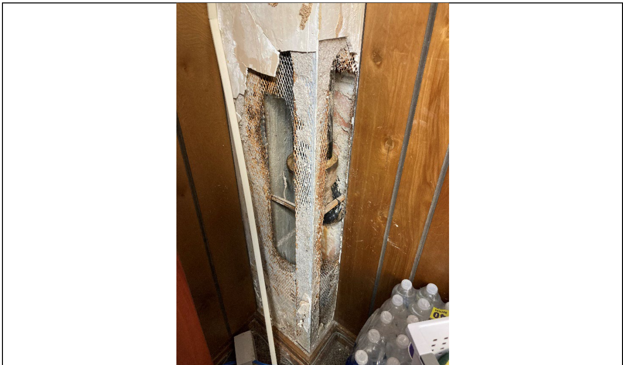
Water damage in courthouse due to water line breaks (basement)
