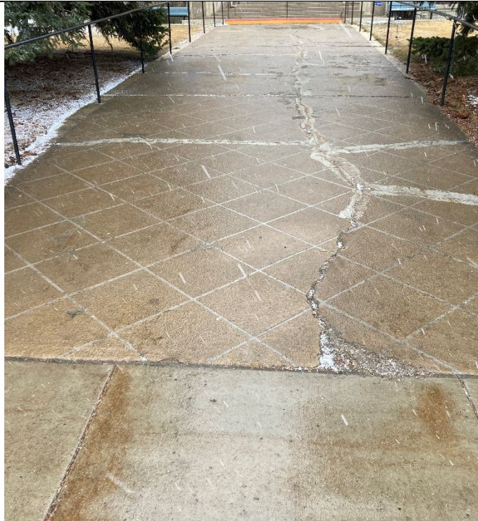
Courthouse entrance concrete cracking
