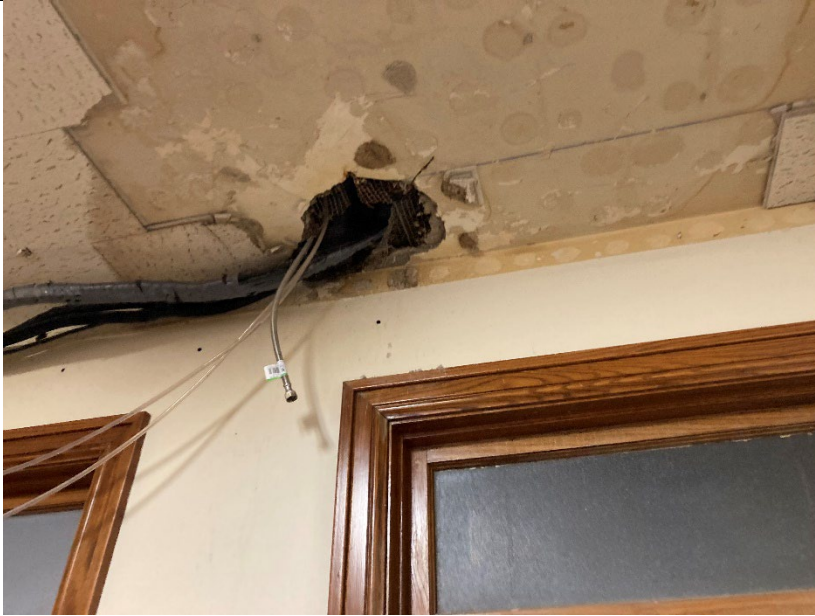
Water damage in courthouse due to line breaks
