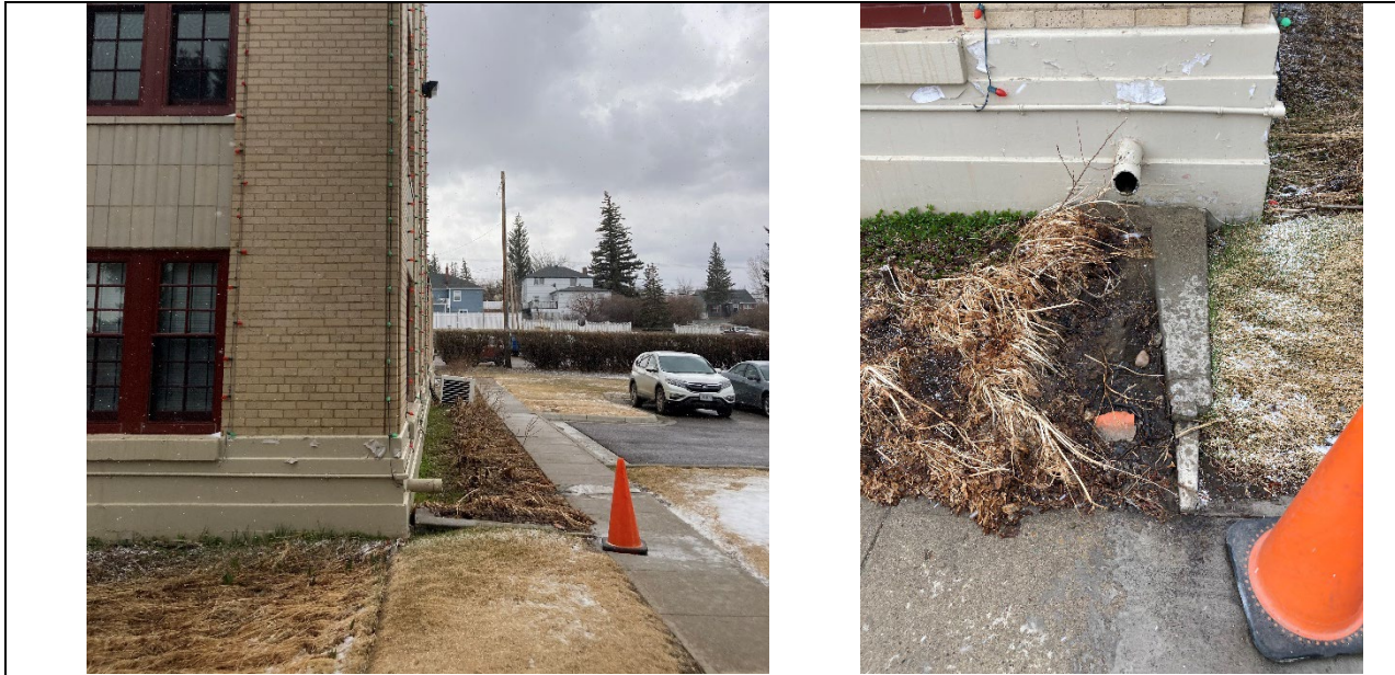
Sidewalk around to accessible entrance – drainage across sidewalk
