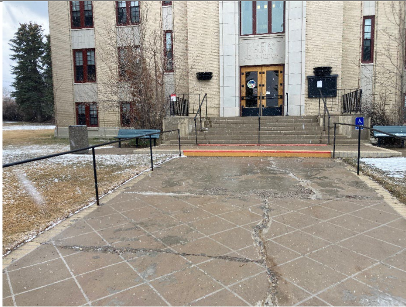
Courthouse entrance concrete condition and stairs
