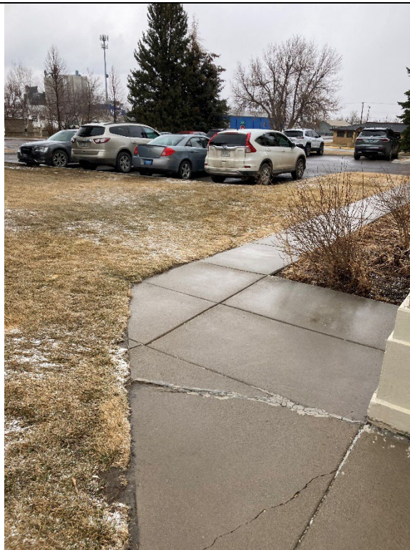
Sidewalk cracking and settlement
