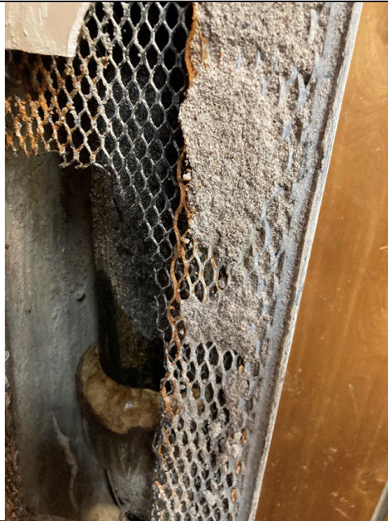
Water damage in courthouse due to water line breaks (basement)
