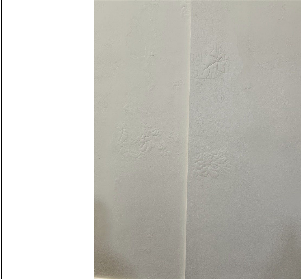
Recently painted wall in courtroom – paint bubbling and cracking
