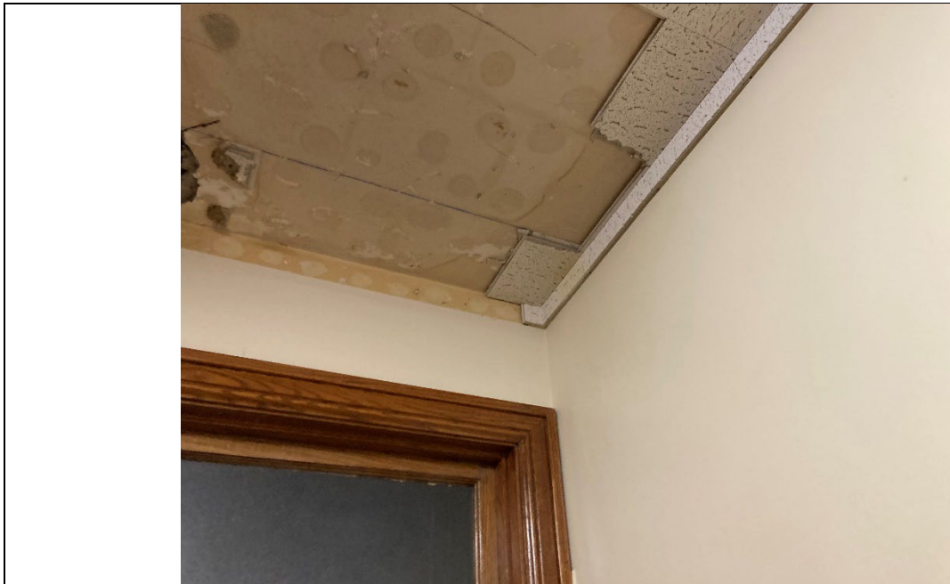
Water damage in courthouse due to line breaks
